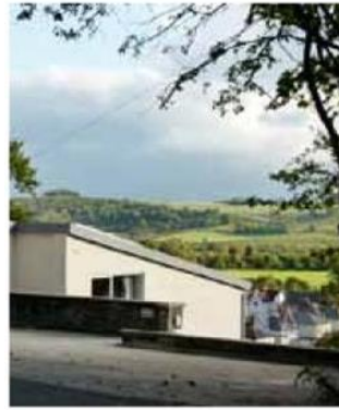
Housing set into the slopes allows panoramic views over roofs
